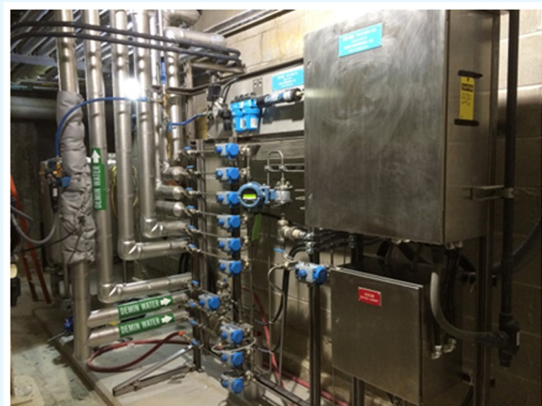
36 FT-NIR liquor analyzer sampling station showing sampling tree and transmission cell.
