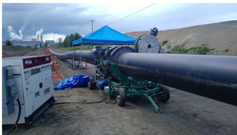
15 Heat fusion of new PE-RT piping system.
