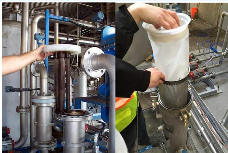
25 Resin trap laterals connected to headplate; resin trap filterbag.
